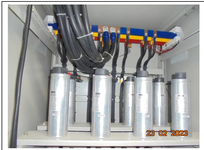
Picture 12: Capacitors Banks Preventive maintenance.
