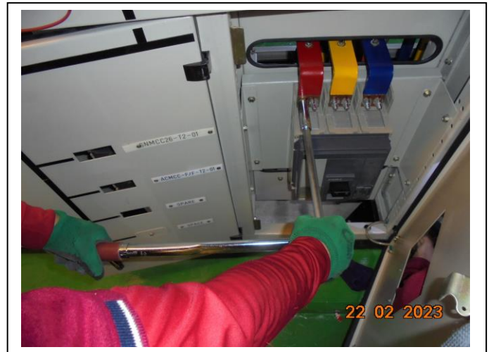
Picture 4: Main distribution board and preventive maintenance.
