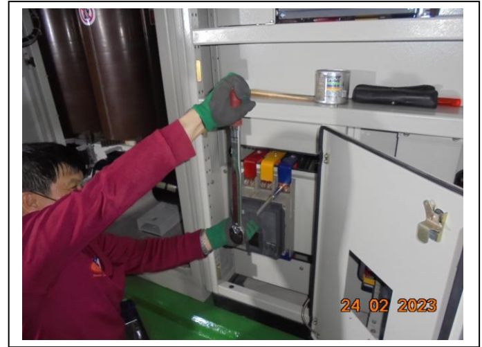
Picture 5: Main distribution board and preventive maintenance.
