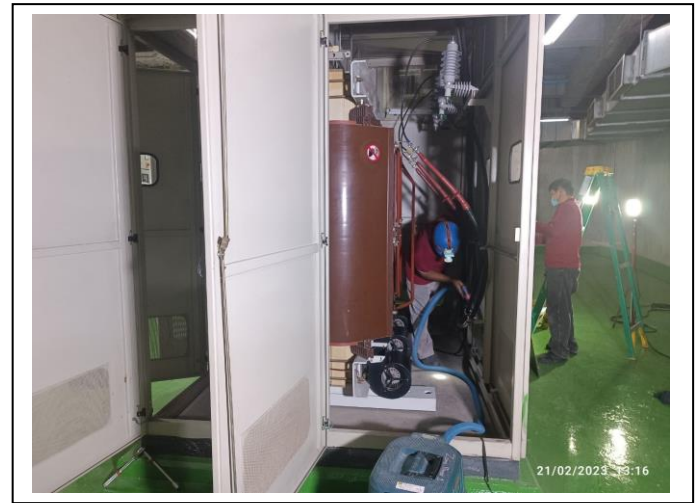
Picture 3: Cast resin Transformer and preventive maintenance.
