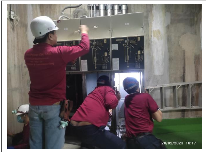
Picture 1: Ring main Unit and preventive maintenance.
