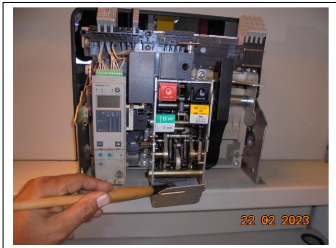
Picture 7: Air circuit Breakers and preventive maintenance.
