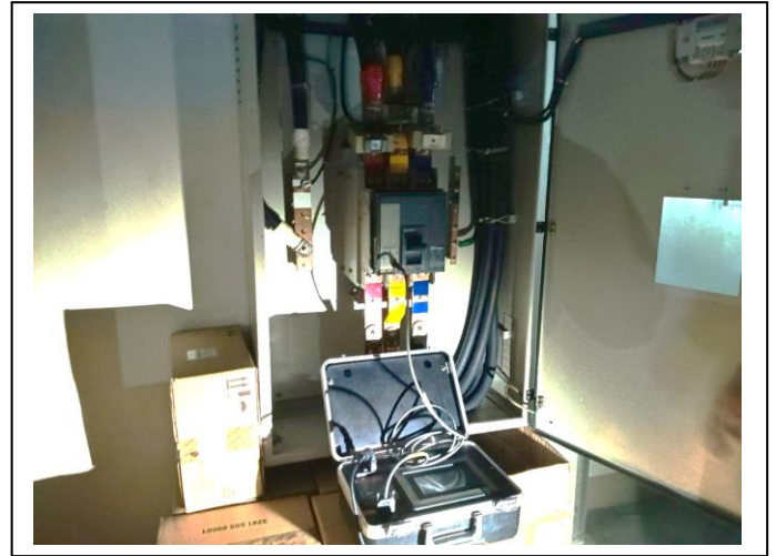
Picture 8: Molded Case circuit Breakers and preventive maintenance.
