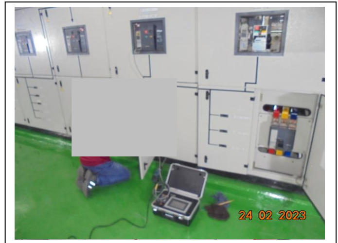
Picture 7: Air circuit Breakers and preventive maintenance.
