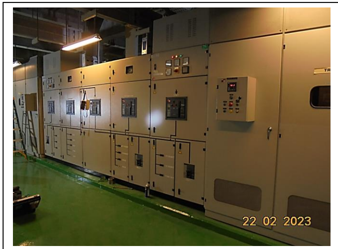
Picture 4: Main distribution board and preventive maintenance.
