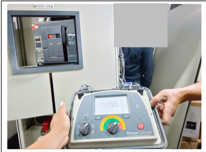
Picture 6: Air circuit Breakers and preventive maintenance.
